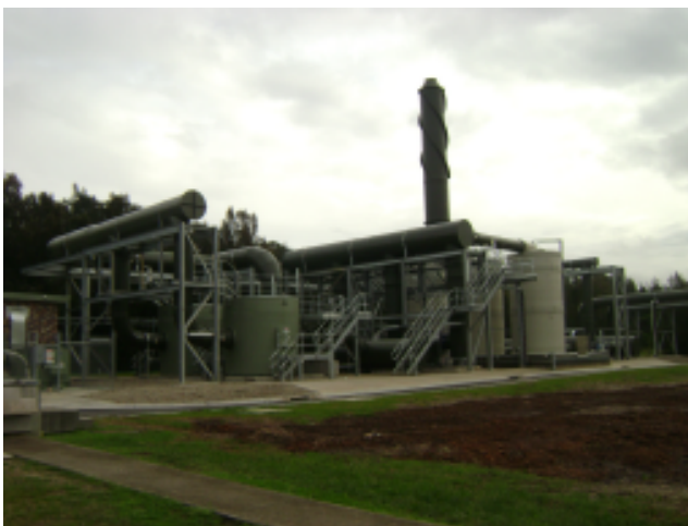
1 st stage Biological Filters with 2 nd stage Activated Carbon Foul Air Scrubbing Plant, Ductwork & Pipe-bridge (Warriewood STP for Sydney Water)
