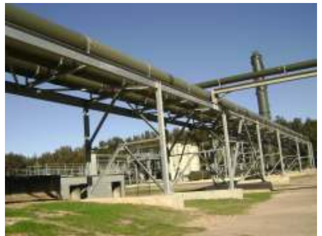
1 st stage Biological Filters with 2 nd stage Activated Carbon Foul Air Scrubbing Plant, Ductwork & Pipe-bridge (Warriewood STP for Sydney Water)
